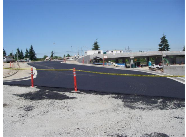
Bus Access Roadway to Bridge #4
