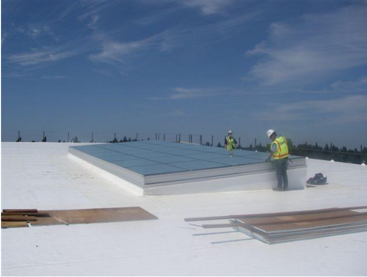
North Escalator Bank Skylight
