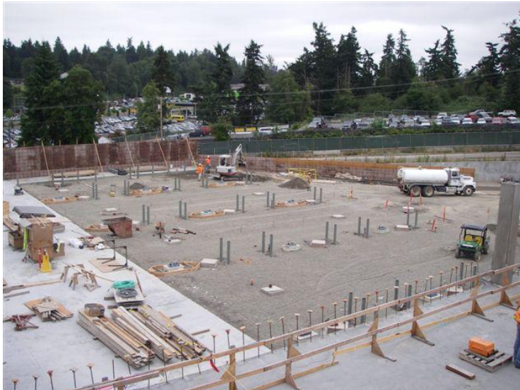
QTA #3 Fuel Island Bollard Installation
